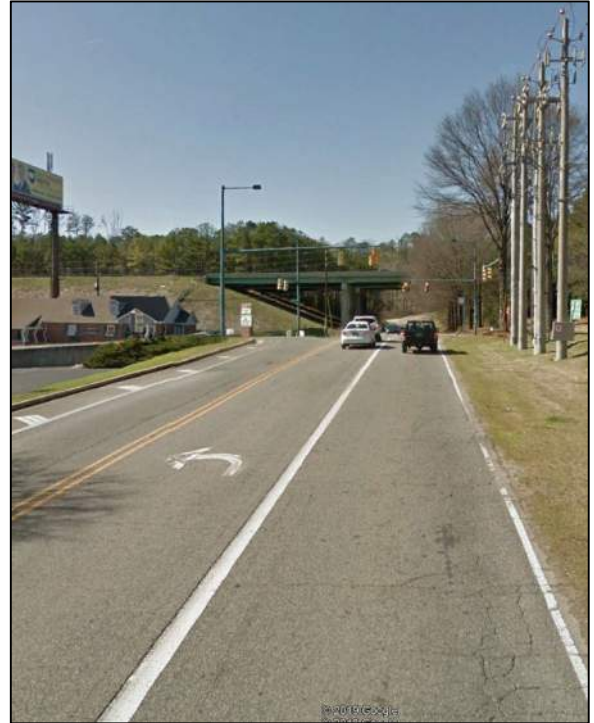
Photograph 2.2: 3-Lane Section at Acton Road Intersection
